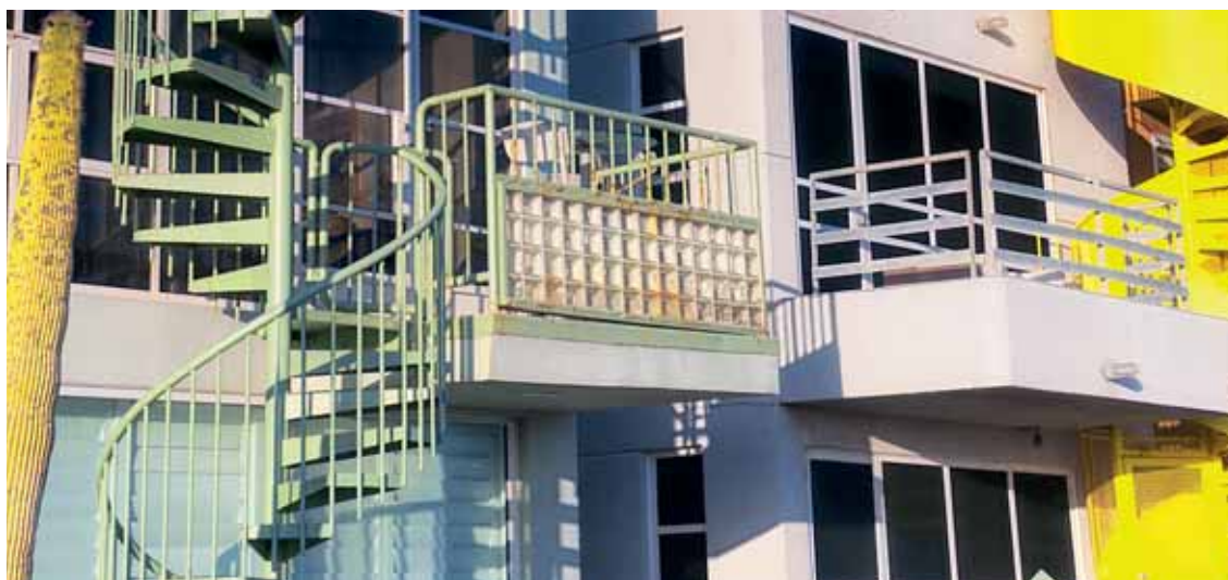
Installation of safety ladders and parapets
