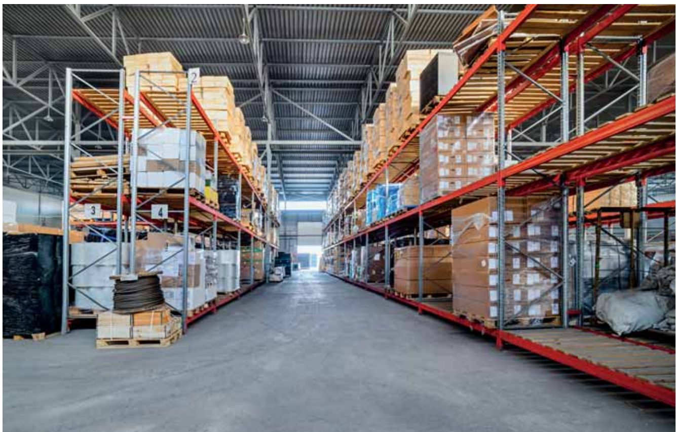
▲ Installation of industrial metal shelving
