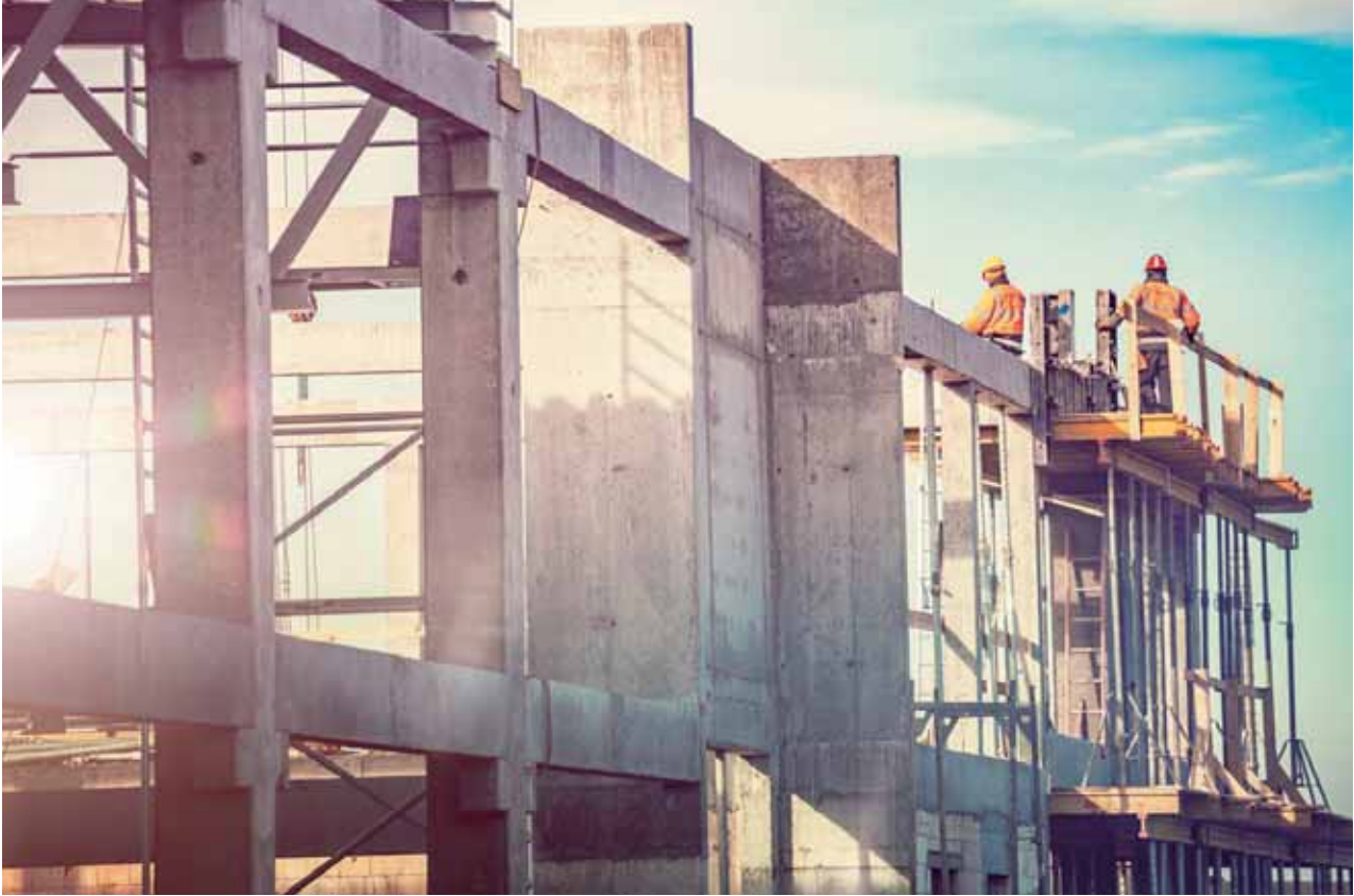
▲ Chemical fixing and construction joints
