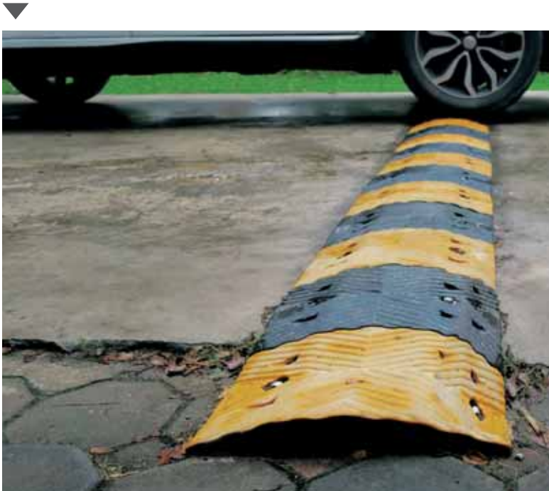
Installation of speed bumps
