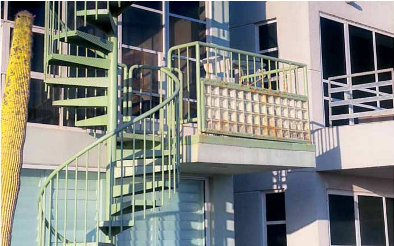
Installation of safety ladders and parapets
