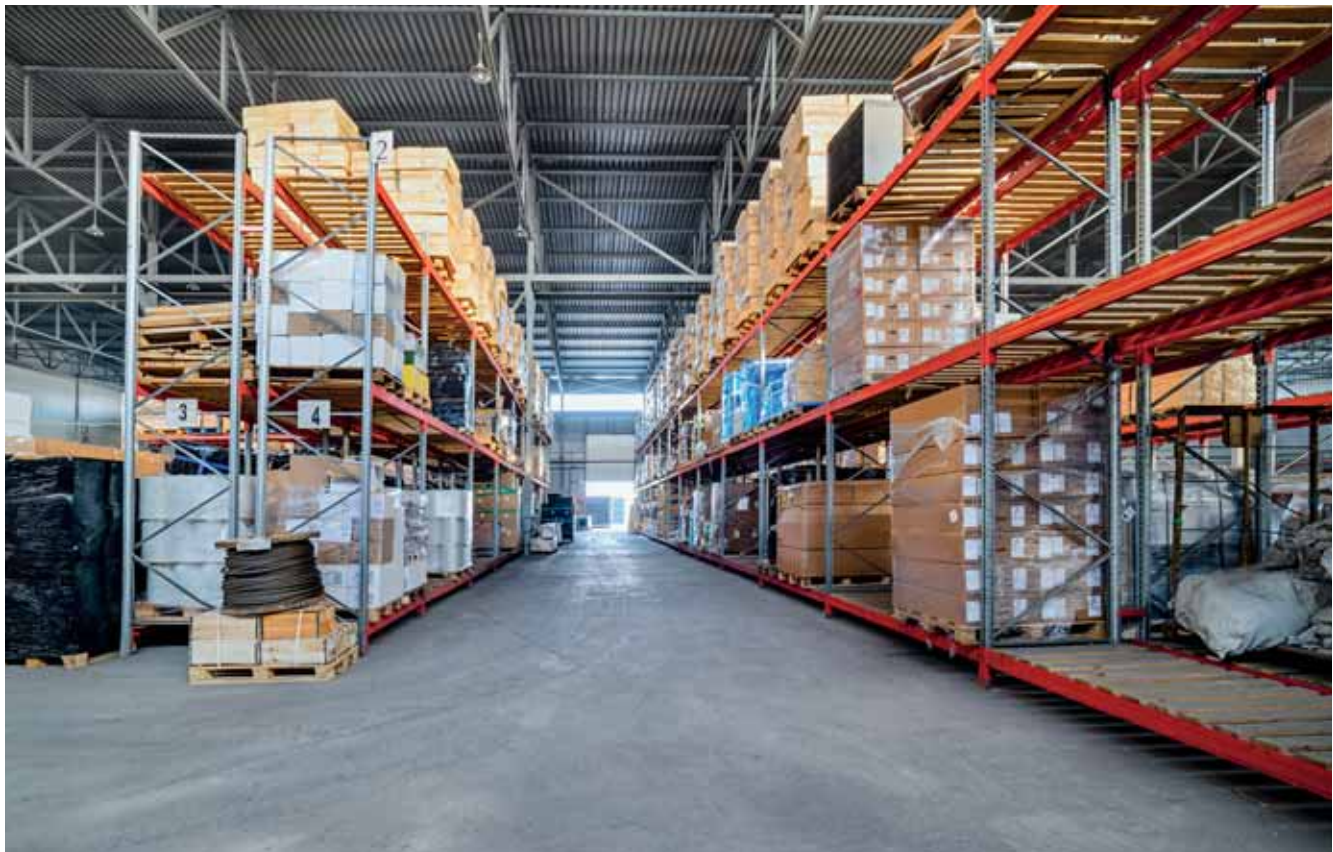
▲ Installation of industrial metal shelving
