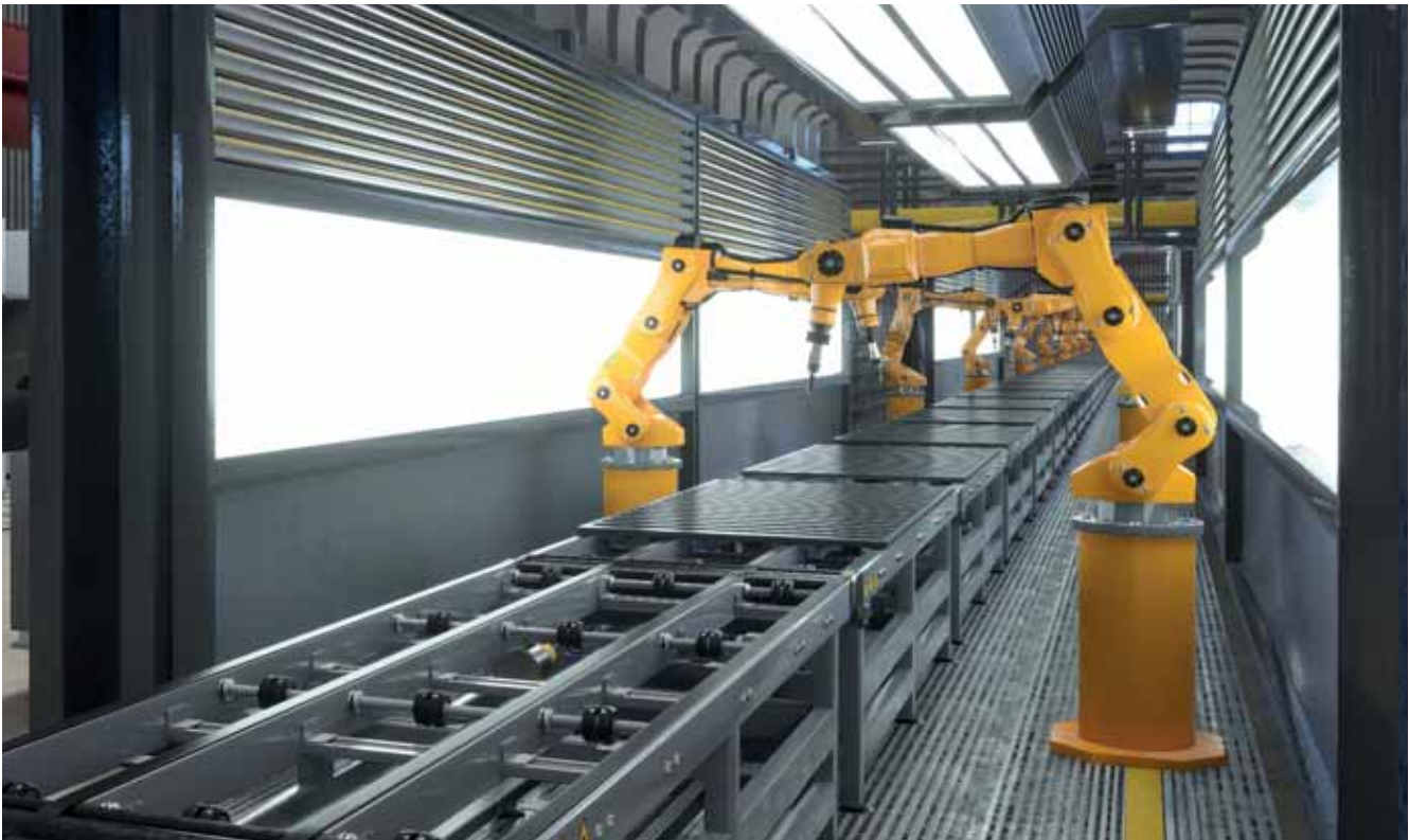
▲ Installation of robotic equipment and assembly line
