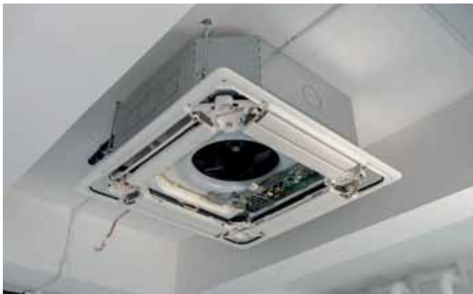
◀ Ceiling air conditioner installation
