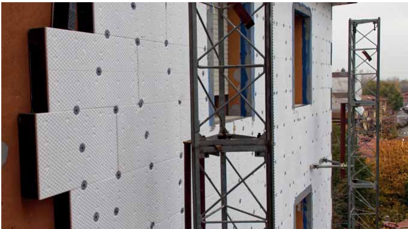
▲ External Thermal Insulation Composite System (E.T.I.C.S.)
