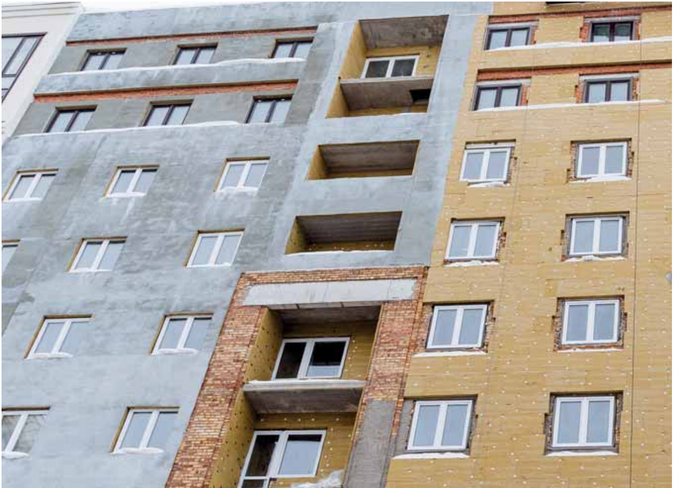
▲ Thermal insulation system application
